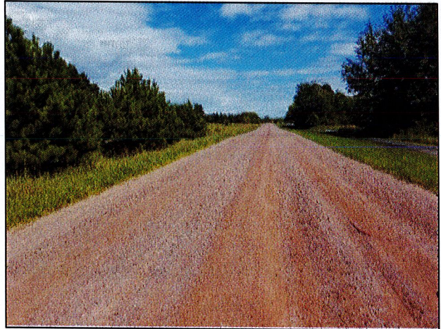
Looking east on 299 th Avenue Northeast
