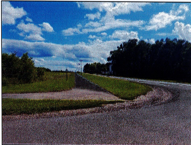
Looking south on Jackson Street Northeast
