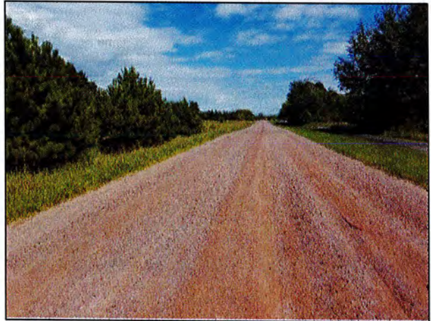
Looking east on 299 th Avenue Northeast
